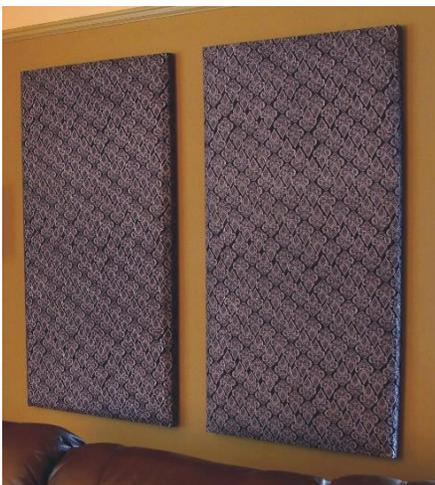
Figure 6: Wrapped Owens Corning rigid fiberglass panels 2'x4'x2" installed on a wall. Fiberglass Insulation Panels, photograph courtesy of, <http://www.amazon.com/Owens-Corning-703-Fiberglass-Boards/dp/B005V3L834>
